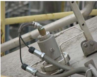
**Twinsburg, Ohio — January 15, 2013** — L.J. Star Inc., the leading provider of process observation equipment, has released a case study that describes how its installation of a [sight glass vessel camera](#) is helping a major U.S. brewery prevent product loss, conserve water, and save time for more efficient operation.
